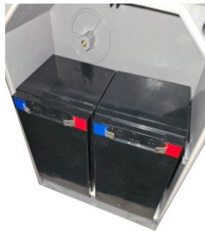
Second battery placed in position
